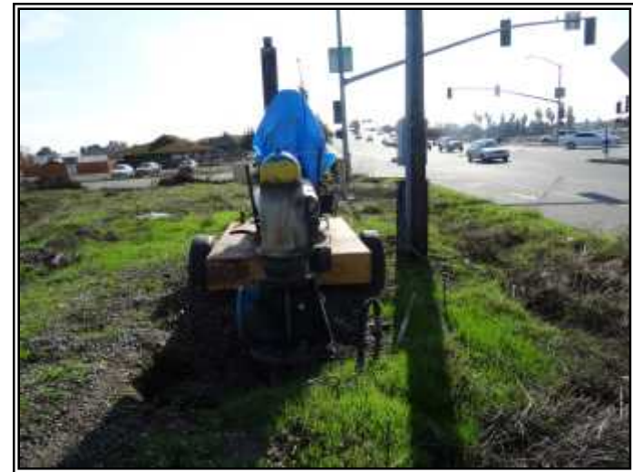
Looking northwest at the irrigation well and portable diesel powered engine on the southwestern corner of APN 033-630-009.
