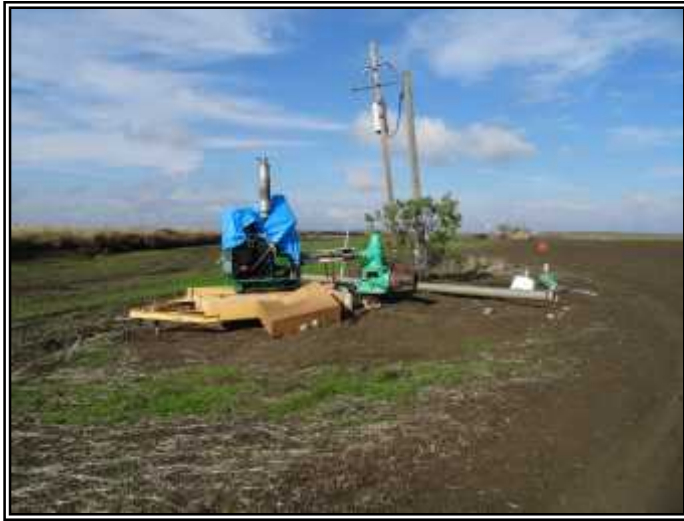
Looking north at the irrigation well and diesel powered engine located on the western portion of APN 033-650-009.
