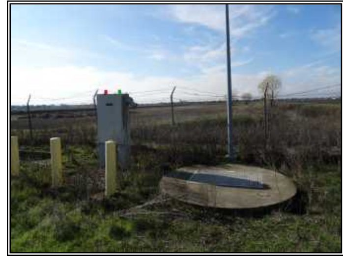
Looking at the an inactive control system associated with the detention basin.
